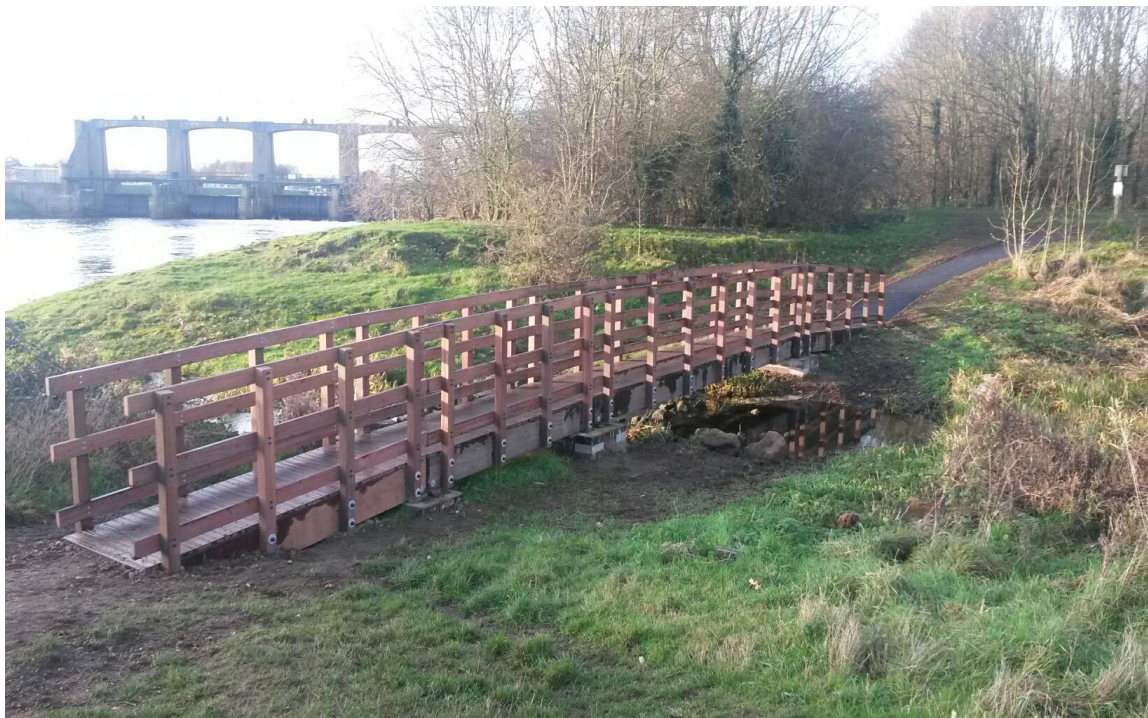
Figure 7: footbridge at Colwick Country Park
