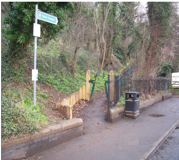
Figure 5: (after) the gate has been removed. To make access for motorcycles and quad bikes more difficult, a motorcycle barrier "A Frame" has been installed
